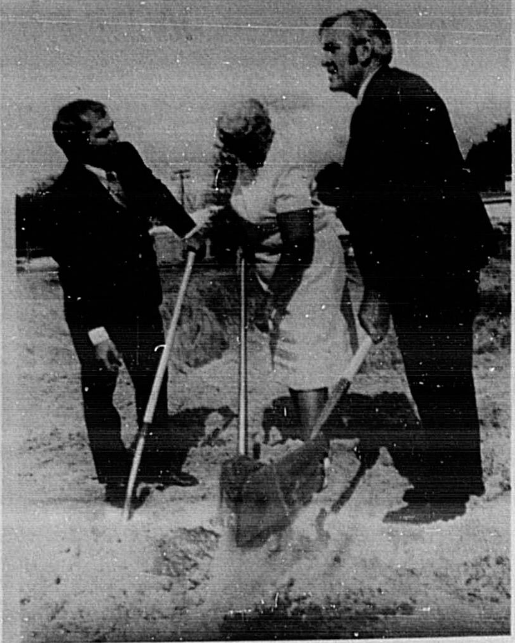
GROUNDBREAKING for the $362,000 city hall being built in Altamonte Springs was held Tuesday afternoon at the site behind the present municipal complex and fronting on Newburyport Avenue. It is expected to be completed before Christmas and work will begin immediately. Welding shovels with gusto are left to right, Councilmen Tom Radloff and Helen Keyser and Mayor Lawrence Swofford. (Ann Riley Photo)
