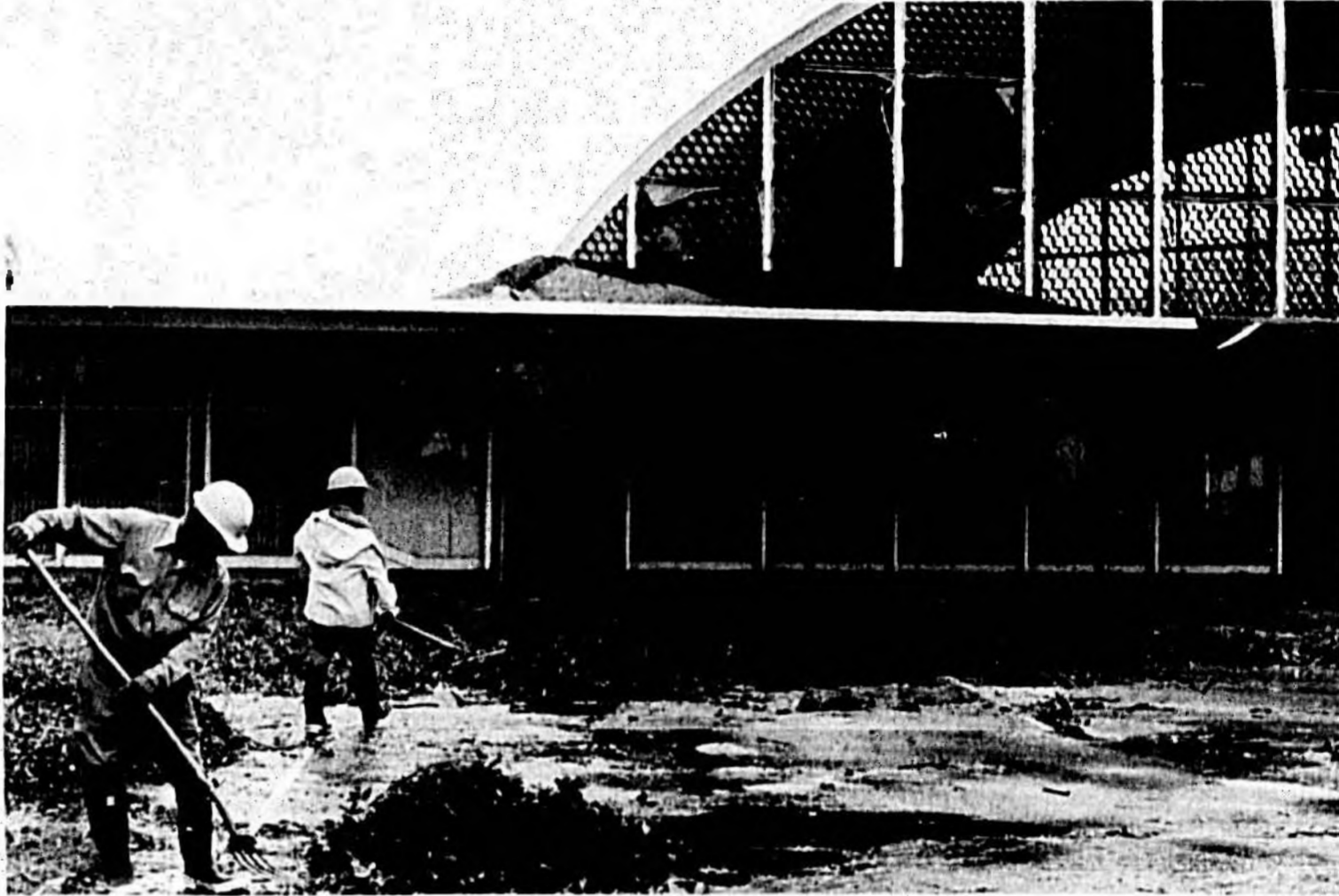
Workers clean up at tornado-damaged Sanford Civic Center
