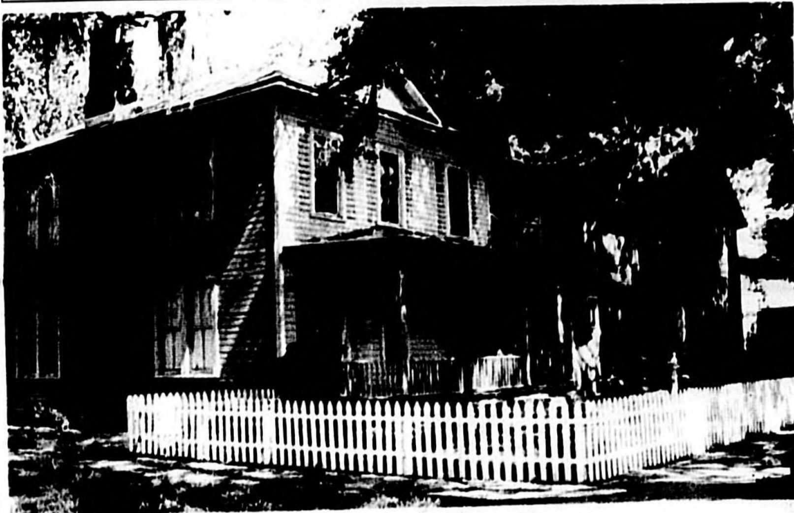
The Myers' Oak Avenue home in Sanford is being restored to its original 1800s beauty.
