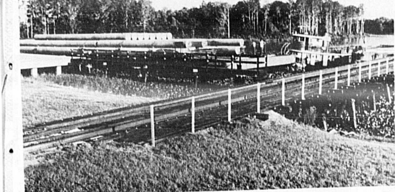
THE FIRST of probably seven or eight barges pulled into the Sanford Port late last night with concrete pilings to be used in the construction of the Orlando East-West Expressway. According to Port Administrator Jim Ryan these barges will be frequent visitors to the area, in a continuing series of barging additional construction materials for major projects in the Central Florida area.
