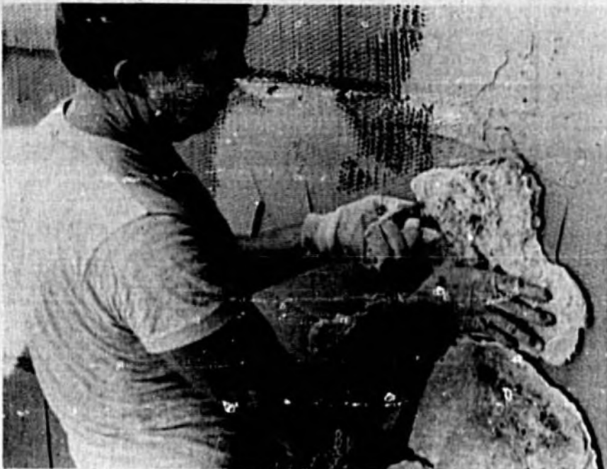
Jack Hopper of DeLand applies Coronado Stone on wall of home in Canterbury at The Crossings in photo above. Photo below shows a finished wall.
