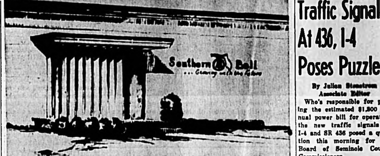
A $135,000 expansion of the Geneva central office of Southern Bell Telephone, due to growth of that area, will be commenced Dec. 1, Manager Robert Shelden said today. A $30,000 building, with $105,000 in new equipment, will be installed adjacent to the present office. Service will be inaugurated June 27.
