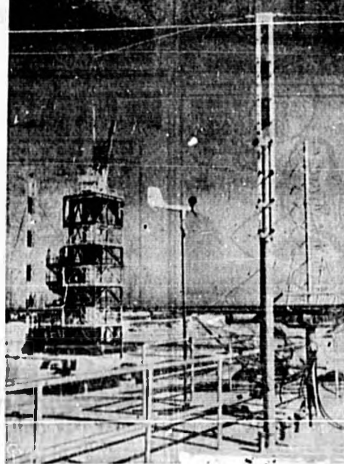
A VIEW OF the earth satellite launching area at the U.S. Air Force Missile Test Center in Cape Canaveral, Florida, as seen from the roof of a blackhouse. The gantry crane at left is used for hoisting rockets on the launching platform. At right is one of the telemetering antennae, which will be used in monitoring performance of the launching vehicles in test flights. (International Soundphotos)
