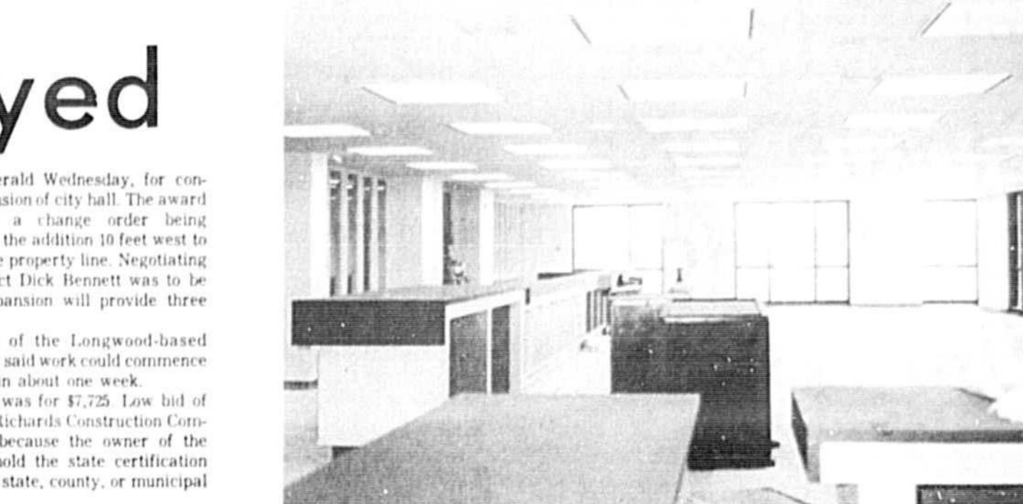
INTERIOR is beginning to "shape up" at the new $19 million Seminole County courthouse, as evidenced in these pictures taken this morning by Herald photographer Bill Vincent Jr. Offices will start transferring from the present courthouse during this month. Top photo shows part of the clerk's office. Lower photo is the main chamber of the County Commission's suite.
