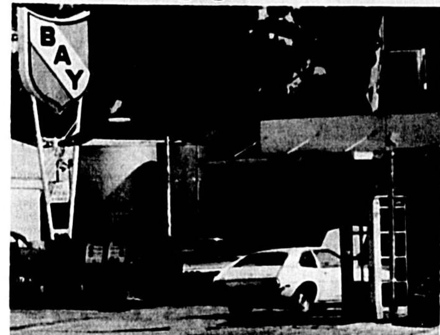
GAS STATION. FUEL STORAGE TANKS SIT ATOP TRAPPED GAS
