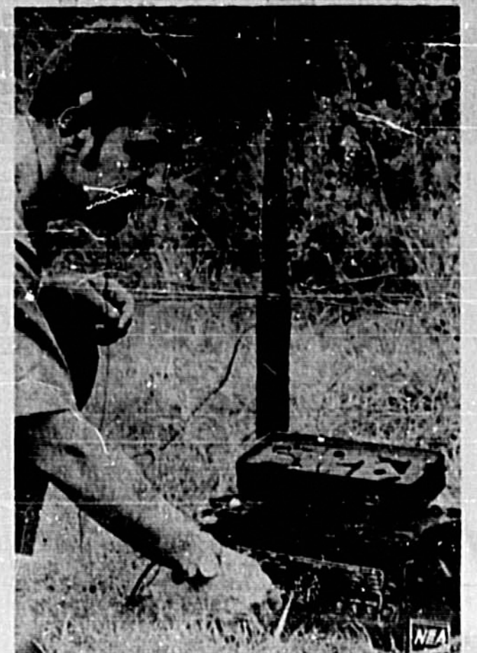
"WHERE AM I?" Aerospace engineer Mike Kearns of St. Petersburg, Fla., knows exactly where he is, thanks to a new device that uses signals from the Navy's navigation satellite system. Completely portable, unit can provide precise location to surveyors and military forward observers.
