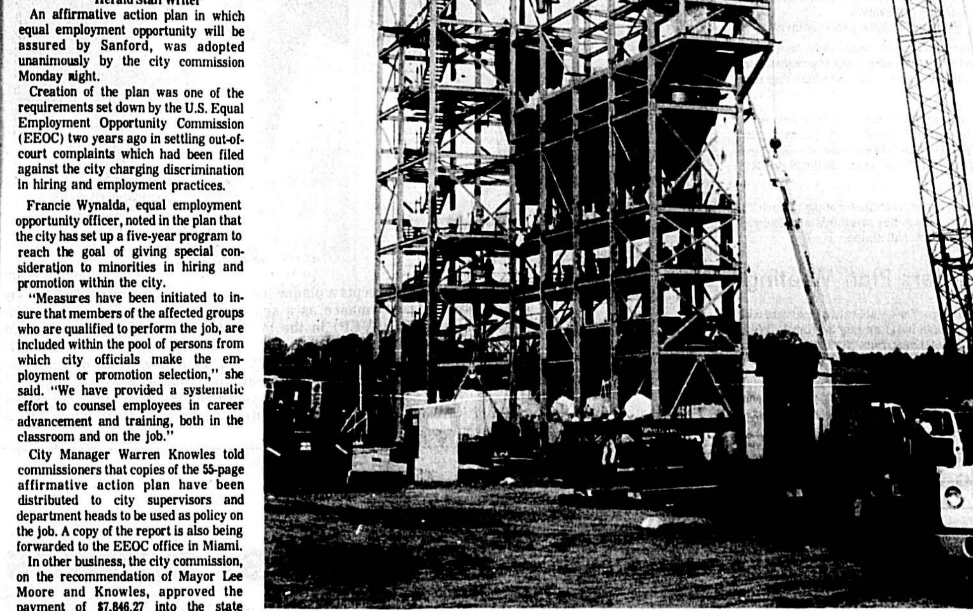
'Oil' mixture plant rises at FPAL's Sanford Station.
