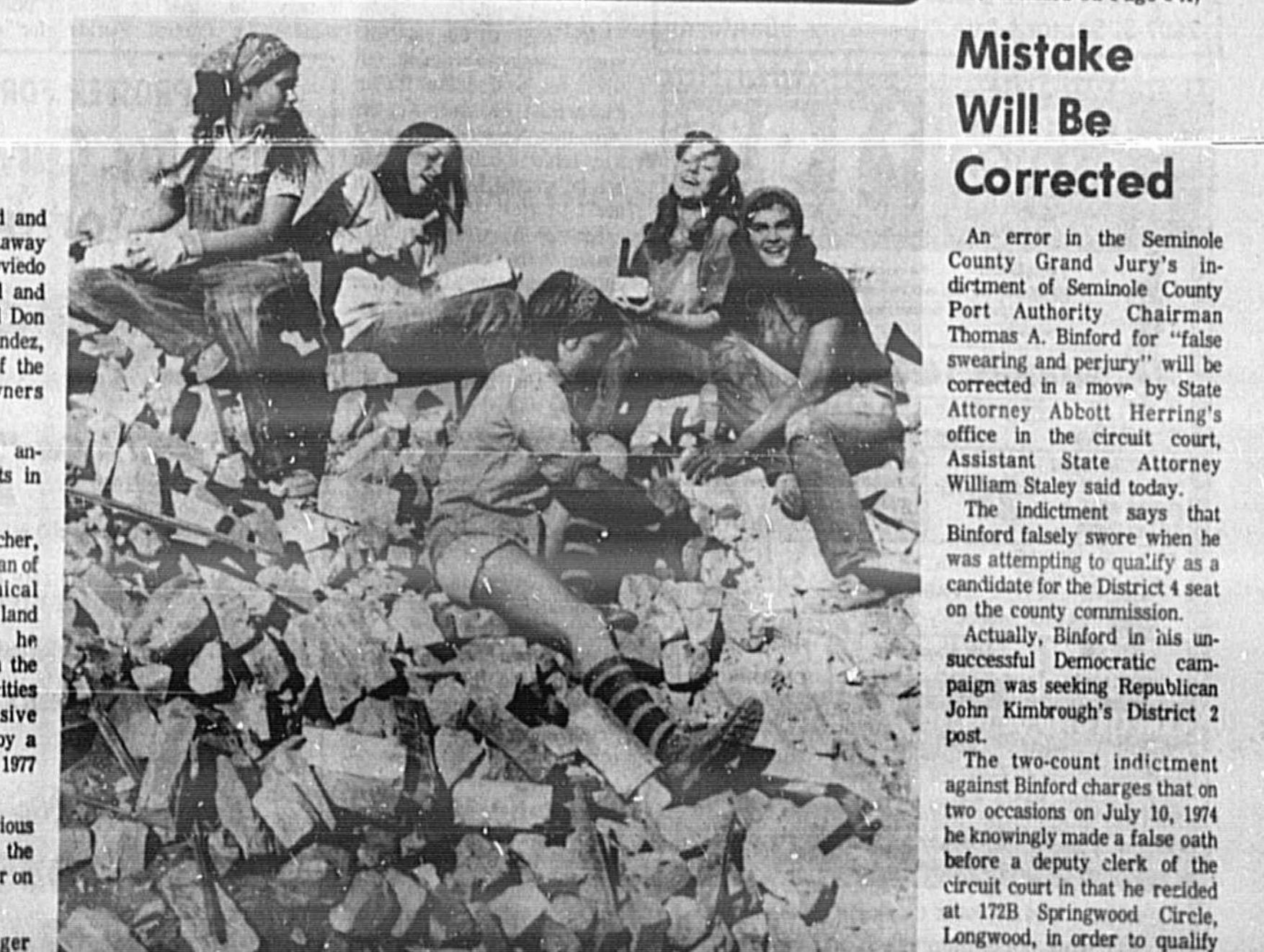
These pretty Crosses High School students have found an unusual way to earn money. They hired out to "chip bricks" at Clowe and Co., where an old building is being torn down to make room for renovations. (Herald Photo by Bill Vincent Jr.)
