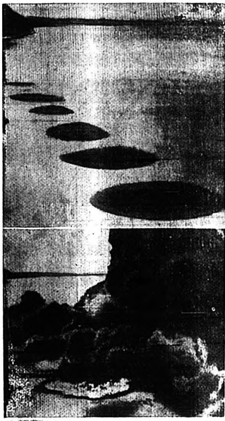
NOW RELEASED is the secret of a British defense against the Nazi invasion that didn't come: the Channel and seas were to be set afire. Underwater pipes were ready, pressured with oil and valves were waiting to be opened at the right moment. The surface oil was to form a thin, inflammable cloud, and the oil-burner sea was to be ignited by shellbursts into a flaming inferno where no ship could live. (International)
