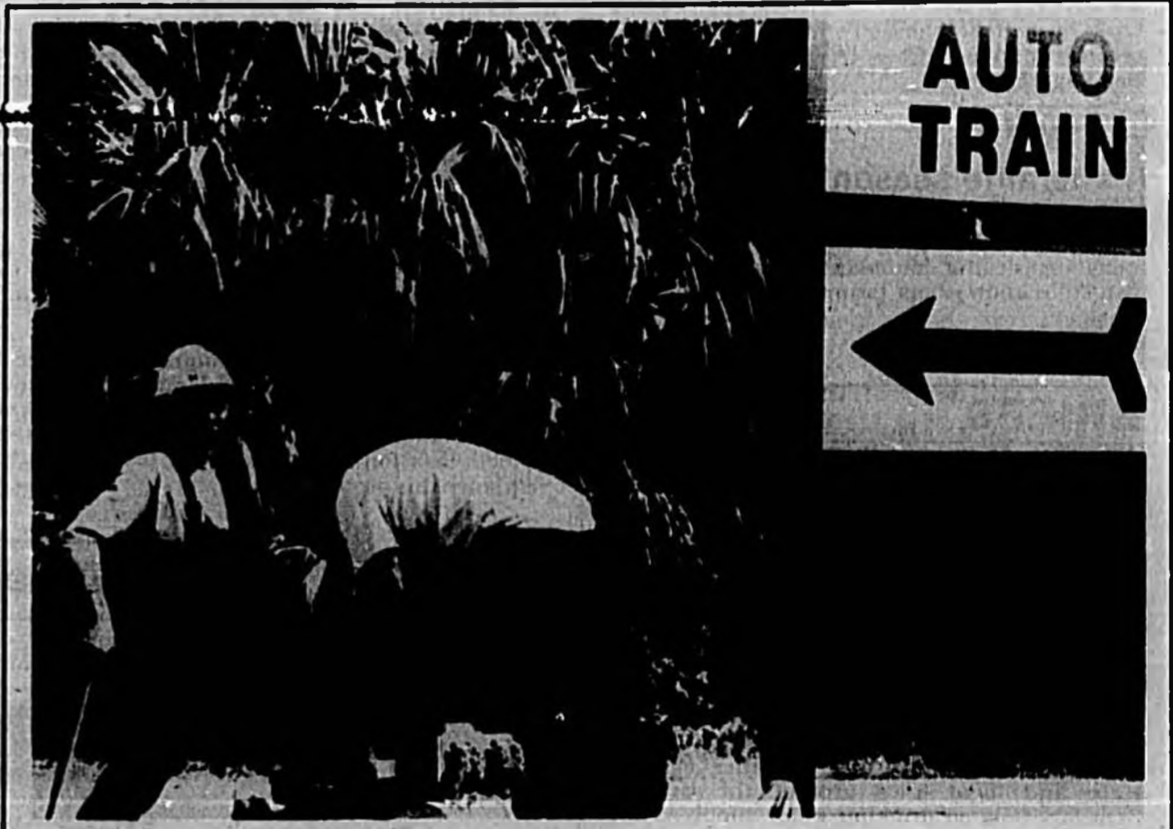
I've been working on the railroad Michael Tsagarakis, the foreman, takes a quick breather, as Bennie Wesley continues work on the reconstruction of the railroad tie wall that is being put in at the entrance of the Amtrak Auto Train facility in Sanford.
