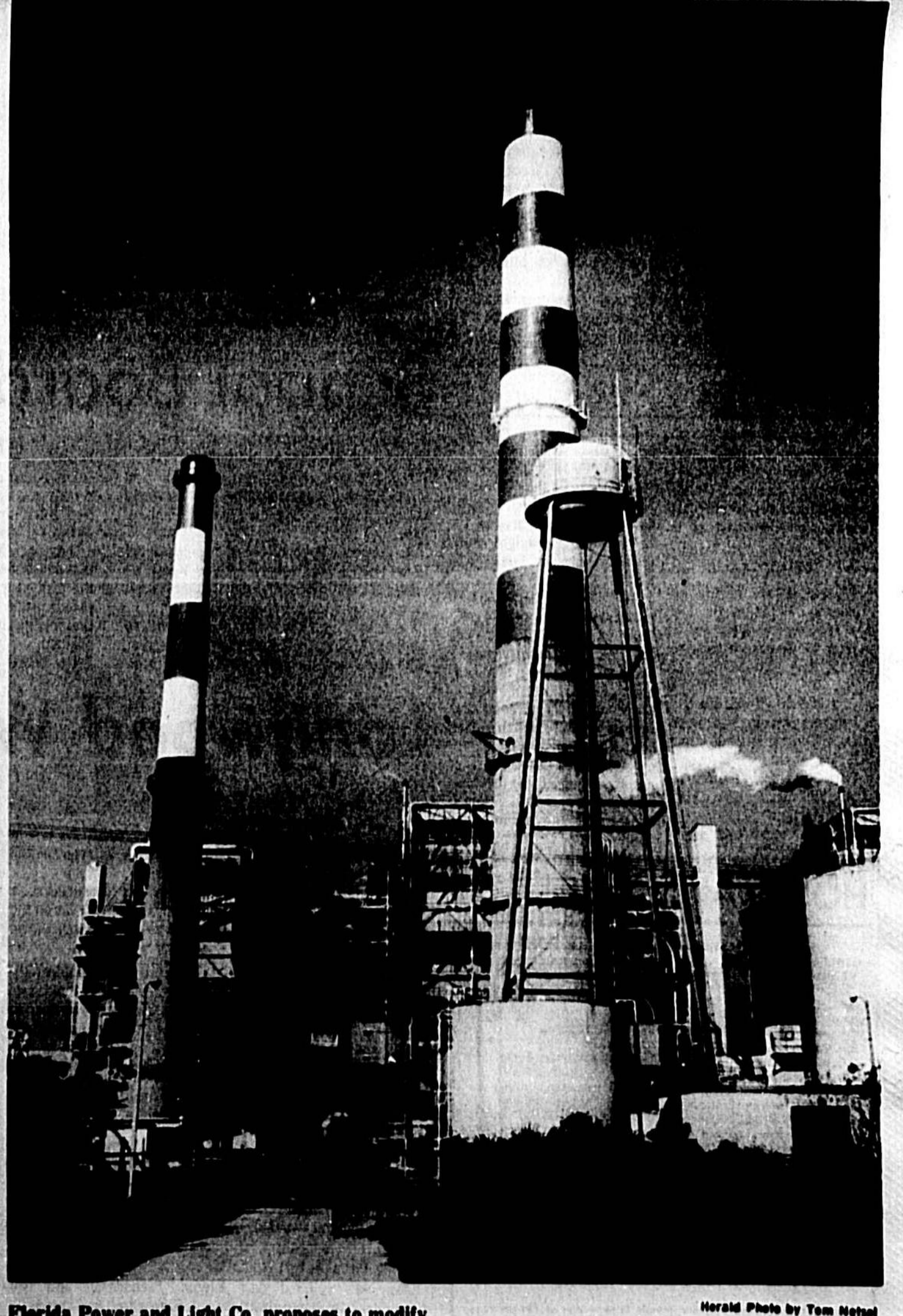
Florida Power and Light Co. proposes to modify the 400-mw plant (shown at right) to burn a unique coal-oil mix.
