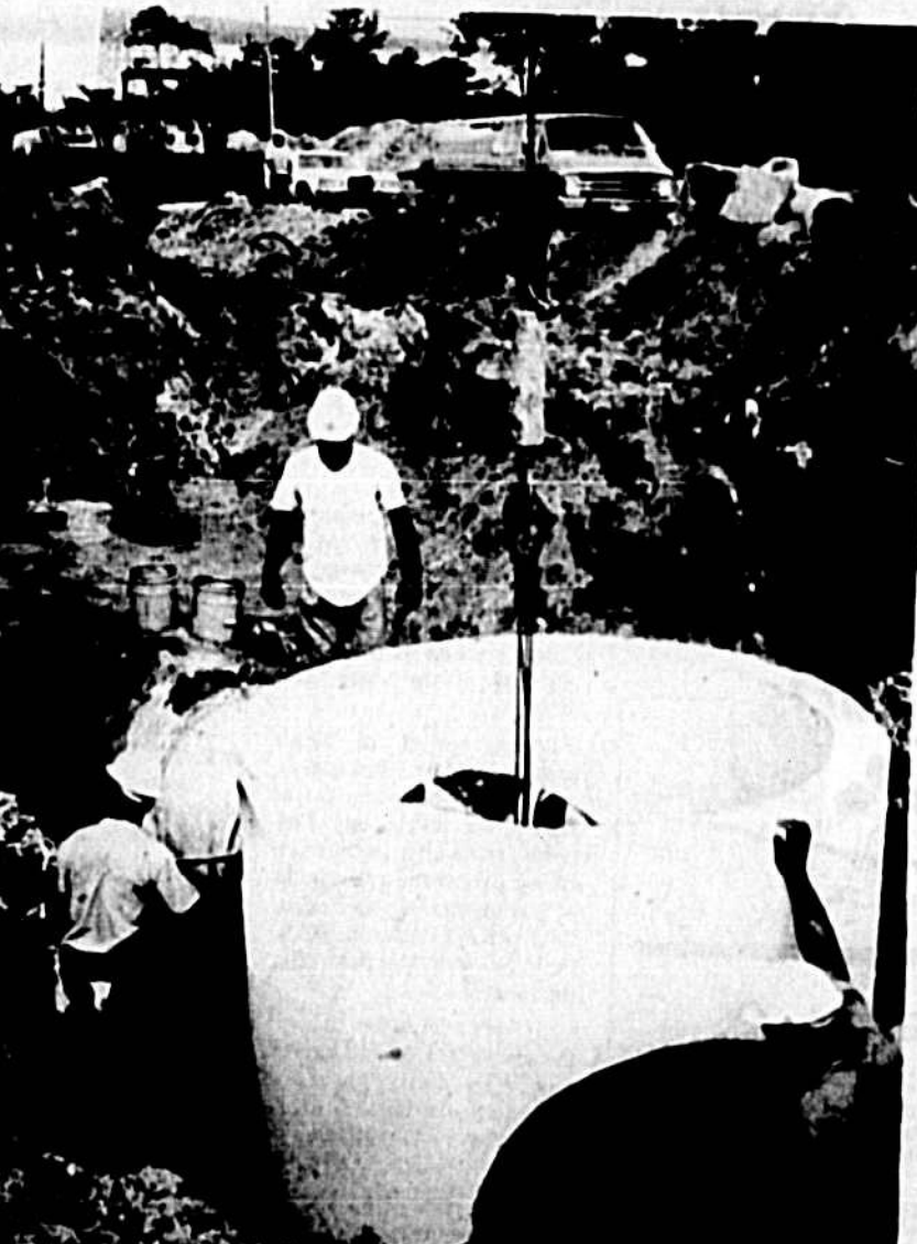
Placement of huge sewer pipes is the work of the day as workers on SR 434 in Winter Springs prepare to begin four-laning the roadway across from Sheekh Golf Club.
