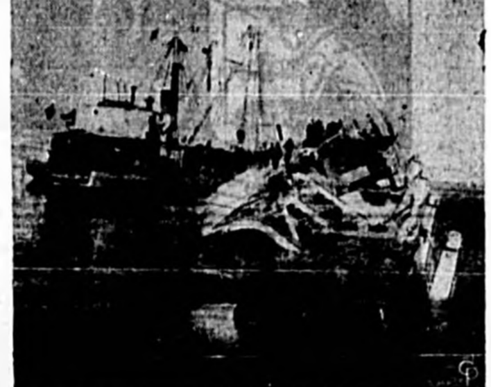
AN ITALIAN SALVAGE CREW on the Squalo ties up to a 8,000-ton LST which was scuttled by bombs acrosswise in the Suez Canal just south of Ismailia. The sunken vessel contains an estimated 2,000 tons of cement. The crew plans to break up the ship with dynamite and then remove the brass sections. The Squalo is one of 14 ships joining in operations of the United Nations salvage fleet. (International)
