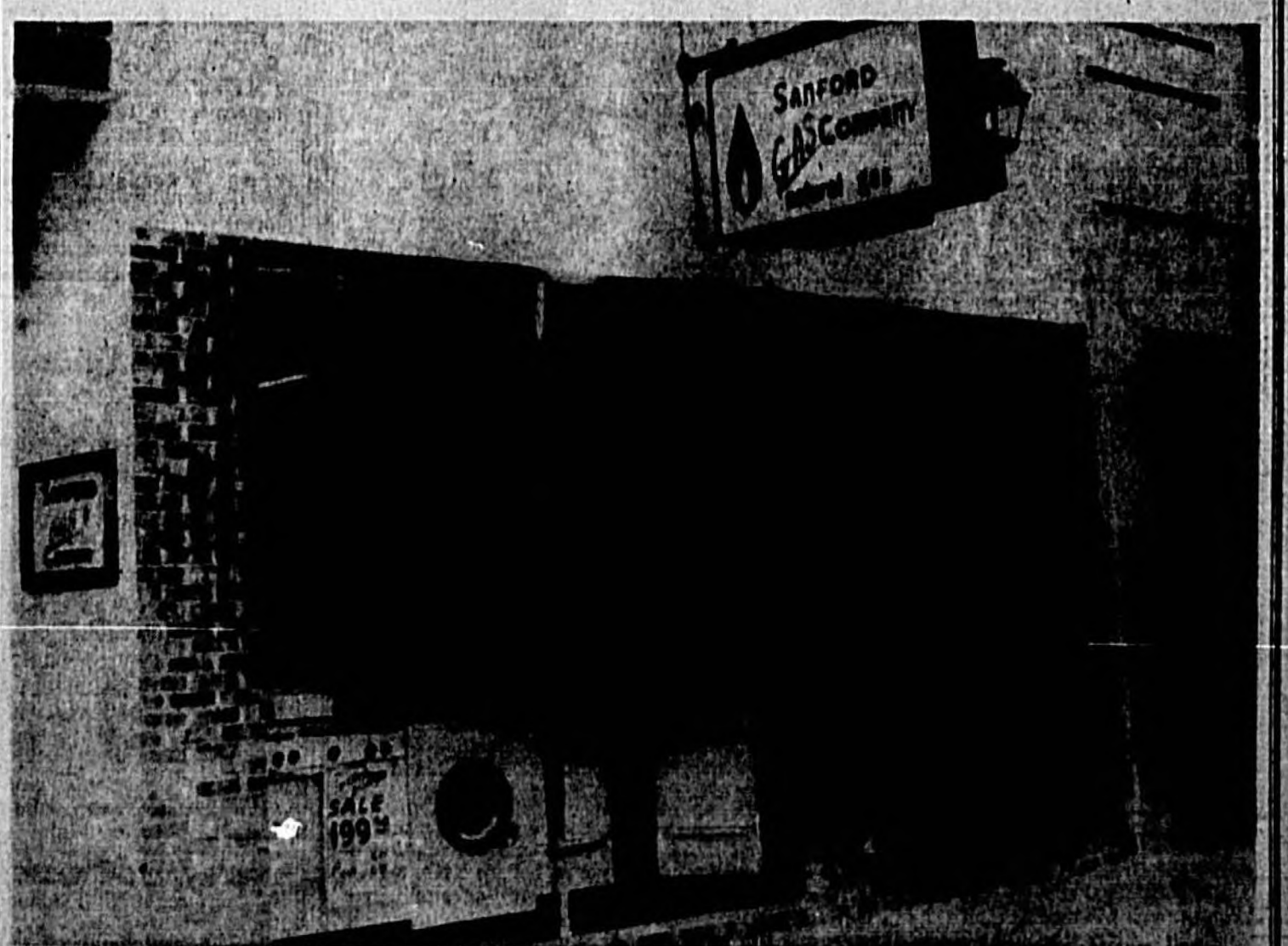
This is SANFORD GAS COMPANY'S new office at 109 West First Street. It is remodeled inside, has new store front, and features a gas lit automatic sign. The gas lamp on the sign burns continuously, day and night. Gas Air Conditioning is now being installed.
