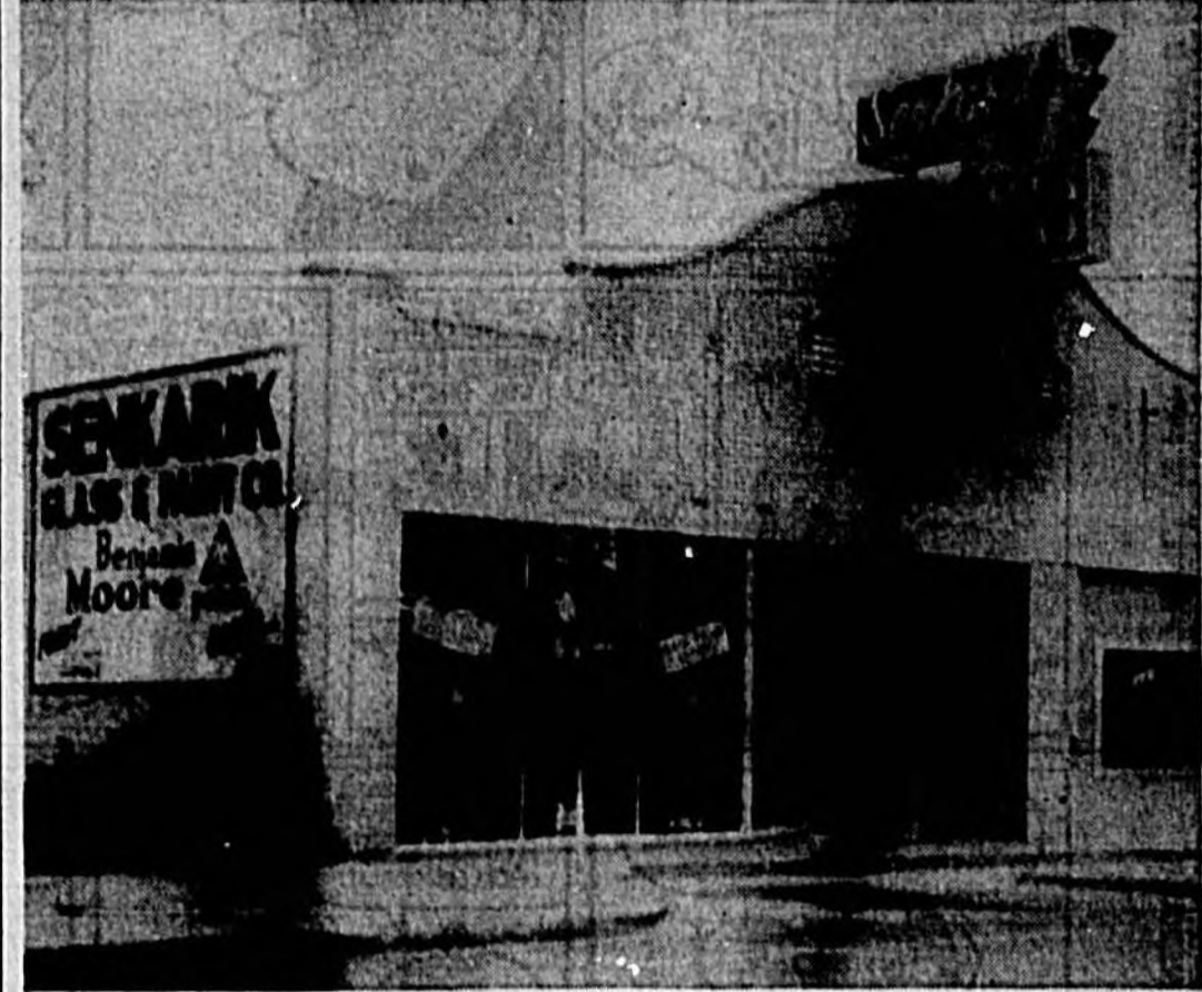
This is the new look of SENKARIK GLASS & PAINT COMPANY , their new store at 210 Magnolia Avenue. The building was completely remodeled, inside and out. Senkarik features paints, glass and glazing, custom manufactured venetian blinds, mirrors, picture frames, and many other decorator items.
