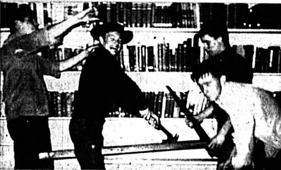
CONTRARY to evidence caught by the camera, these four Geneva youths, Perry Thomas, Leo Ford, Turby Kinniard and Jack Romans (left to right) are "all business" most of the time as they build additional shelves for the new library to hold books which are being donated regularly.
