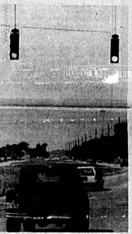
New traffic signals at west state Road 46 and Airport Boulevard.
