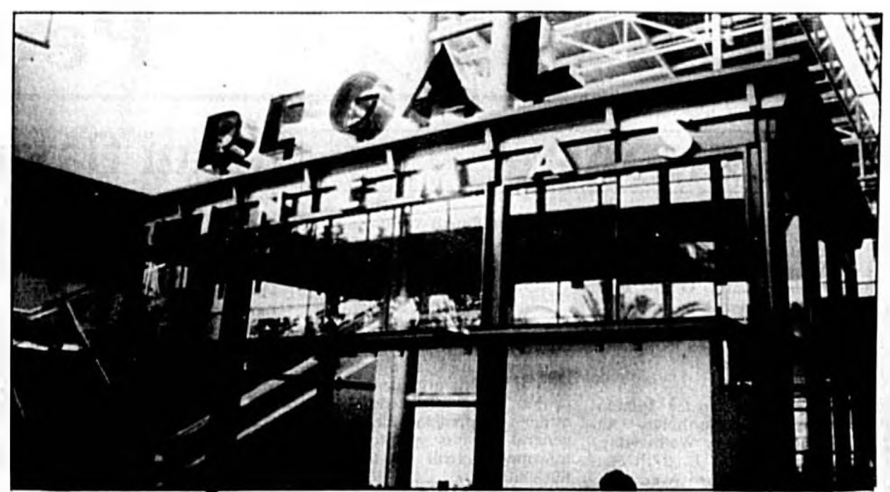
The Oviedo Marketplace Regal 22 has postponed its grand opening due to wiring problems.
