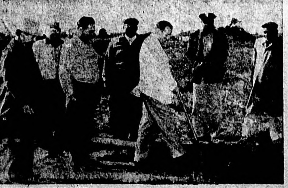
THE FIRST SPADE OF DIRT was turned on the 50-acre recreational area in Goldsboro Friday by Supt. of Schools R. T. Milwee. Others taking part in the ceremony (left to right) are: County Commissioner Fred Dyson, School Maintenance Supervisor C. C. Howard, City Commissioner John Krider, Herbert Cherry, Chairman of Committee of Colored Citizens for the project, Leroy McLendon and James Hagan, committee members. (Staff Photo)
