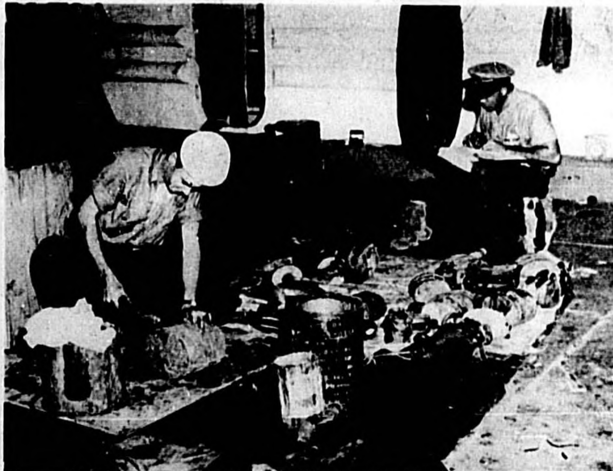
This isn't a cushion on a space ship, but an aluminum seal over a gun turret on a war craft of Florida's Silent Fleet. A crew member is taking a reading of the interior humidity.
