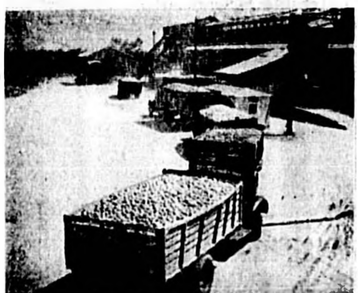
When Florida's many citrus processing plants begin to run at full capacity, large semi-trailers crowd the receiving yard, sometimes in long lines, as above, waiting their turn to back down the incline to the receiving bins where a loosened tail gate sends a golden stream into the first phase of the processing.
