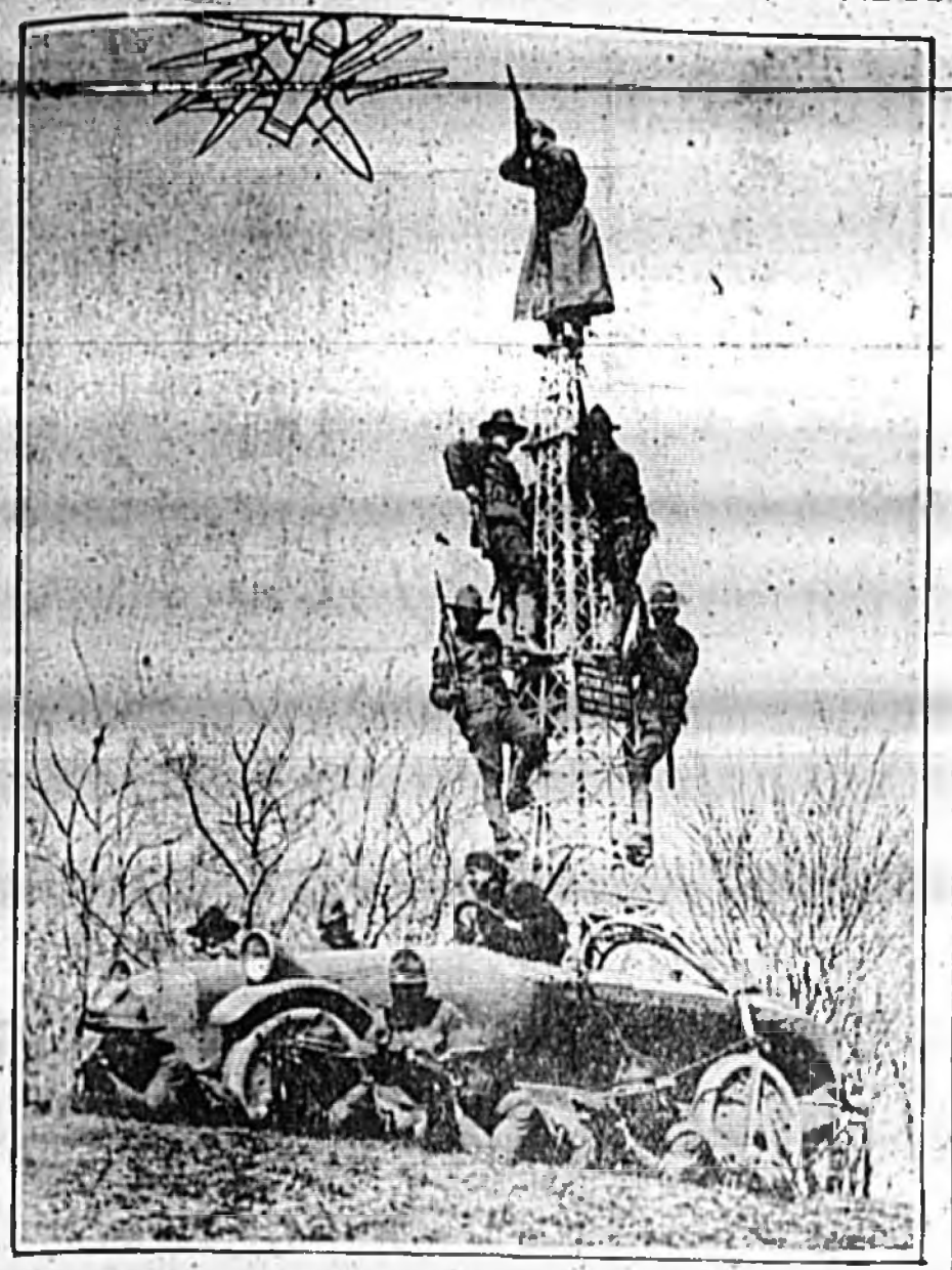
Photo by American Press Association. This newly invented armored car is fitted out with a wireless and observation tower that resembles a miniature Eiffel tower. The tower is hinged and breaks in two.
