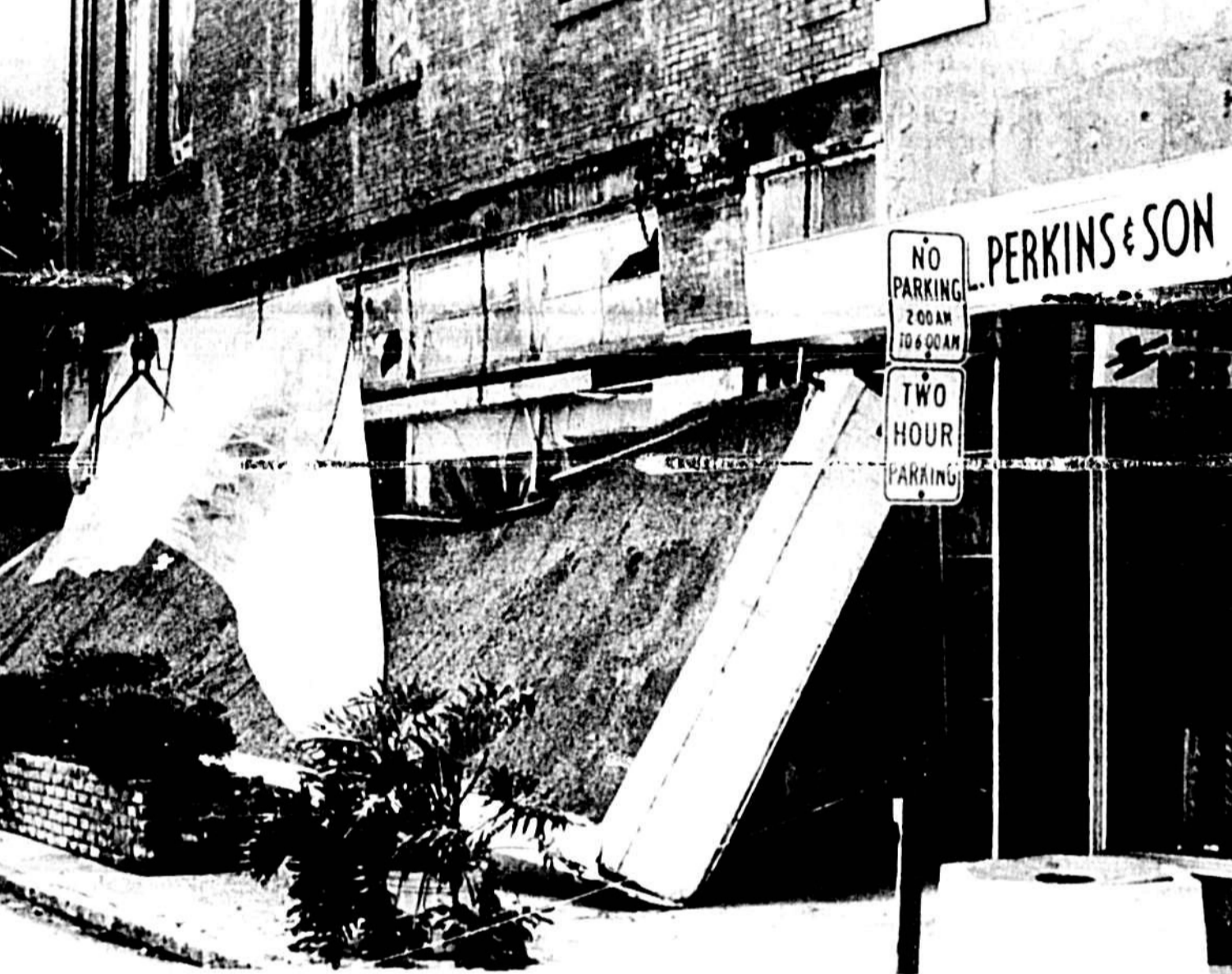
THE CANOPY CAME DOWN Four workers escaped injury Thursday when the canopy they were standing on above the first floor of Garrett's Department Store at 200 E. First St. in Sanford collapsed. Portions of the canopy smashed the front window of the building. Total damage was estimated at $18,000.
