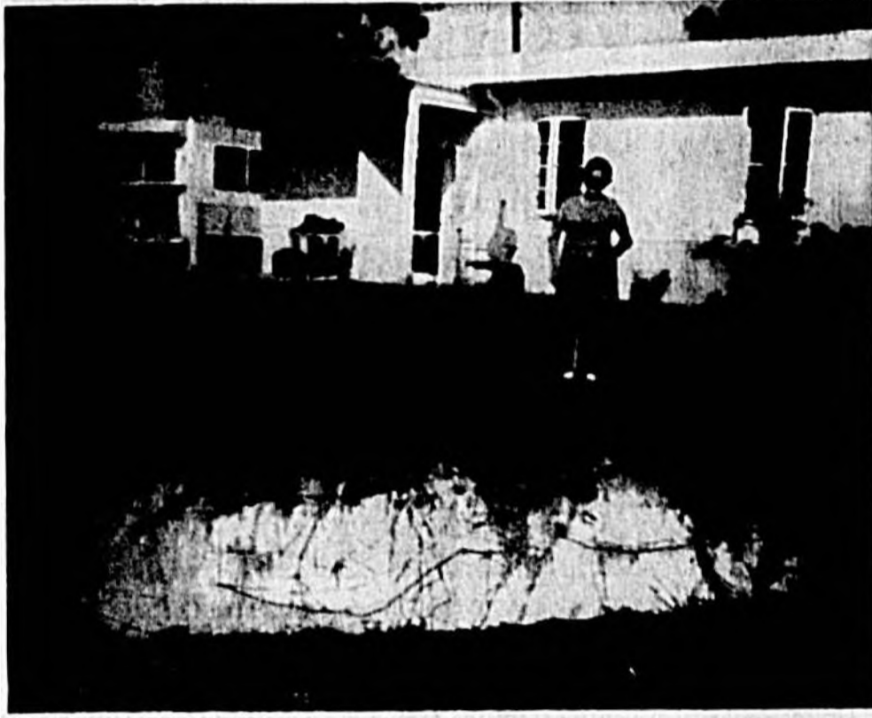
LATEST SINKHOLE to form in the Casselberry-Fern Park area developed to a depth of some 10 feet early Wednesday morning in the backyard of Mr. and Mrs. Garnie Bessinger on Fern Park Boulevard. Mrs. Bessinger, shown here surveying the damages, says that she and her husband are keeping a "wary eye" on the situation. (Herald Photo)
