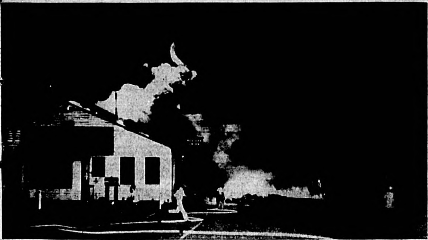
FLAMES AND SMOKE BOILED FROM the burning Sanford State Farmers Market early this morning. Flames can be seen as they leaped across the paved area into the adjoining market building. (Photo by Bergstrom)
