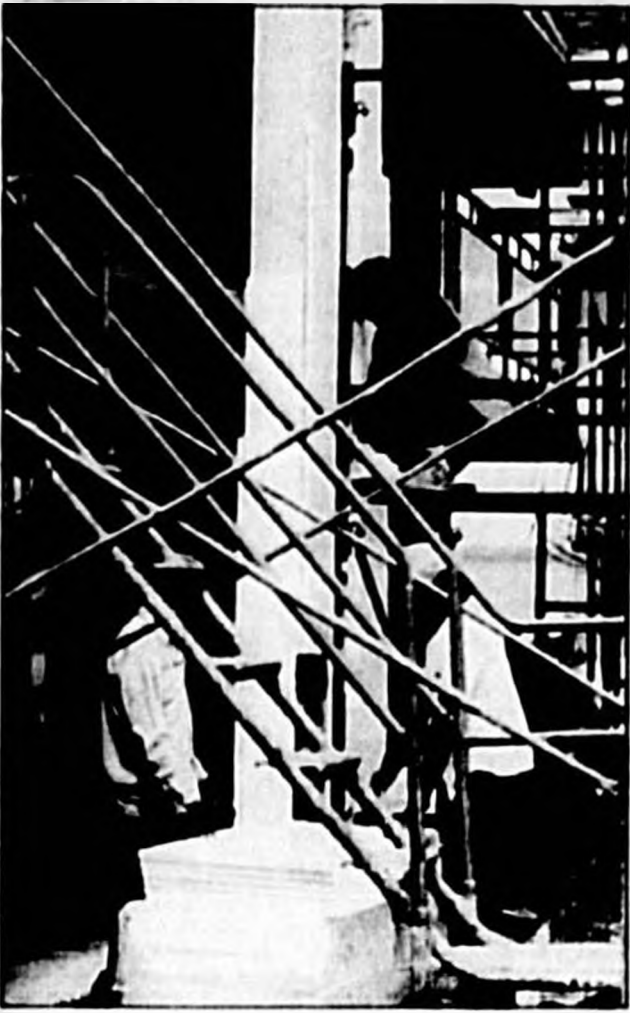
The Marina Hotel is currently under re-construction. The project is being conducted by contractor ENCON of Longwood. Pictured, Lois Garcia puts up sheetrock for exterior columns and Pedro Monos and Pedro Man help him.
