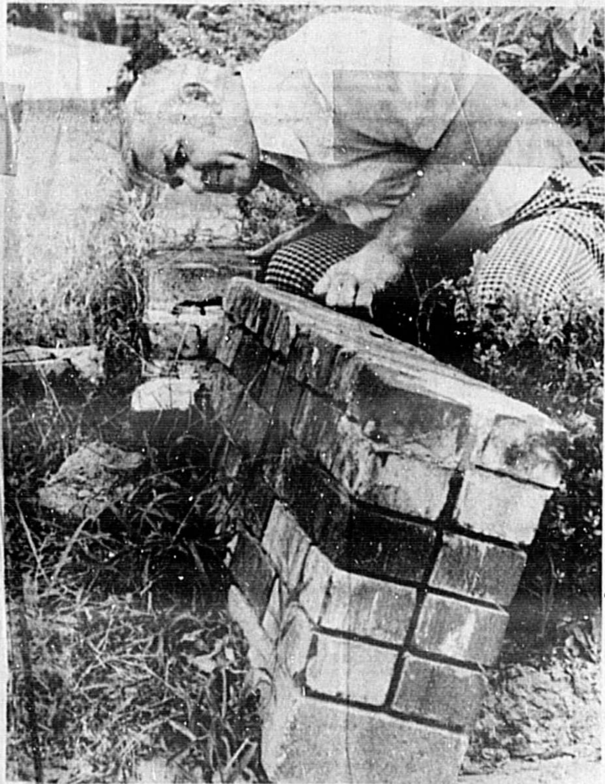
Former Mayor Lawrence Swofford of Altamonte Springs examines one of the walls at his Lake Florida home damaged when sewer lines were installed.
