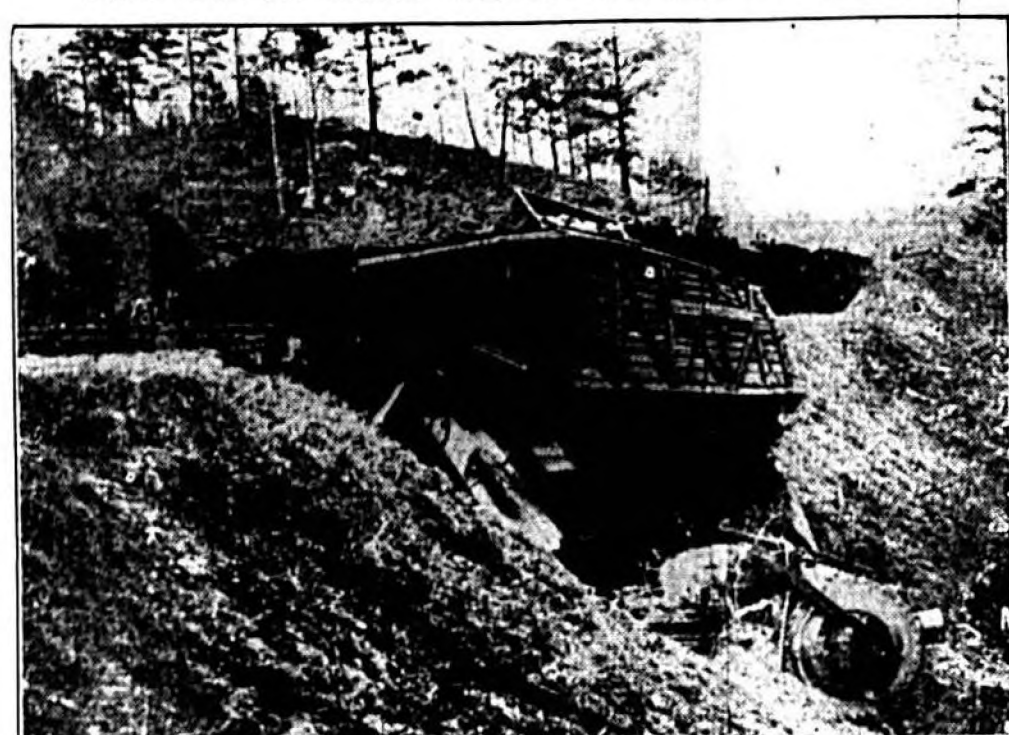
Two trainmen, brakeman J. M. Brown and fireman Frank Kenamer, were killed near Maxwell, Ala., in the wreck of a freight train caused by flood water. The locomotive, which can be seen buried in the ravine, and a number of cars plunged from the track undermined by the torrents. (Associated Press Photo)
