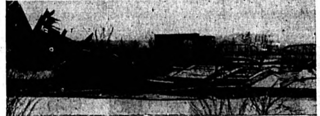
Torrential rains and tornadoic winds that struck almost simultaneously in sections of Florida, Alabama and Georgia caused 18 deaths and did uncounted property damage. At the top is a view of an Alabama Coast Line passenger train that was derailed by a washout near Panama, Ala. The picture below, made after a tornado swept over the countryside near Cottonwood, Ala., shows the ruins of a barn in which John Condry and his wife were injured. (Associated Press Photos)
