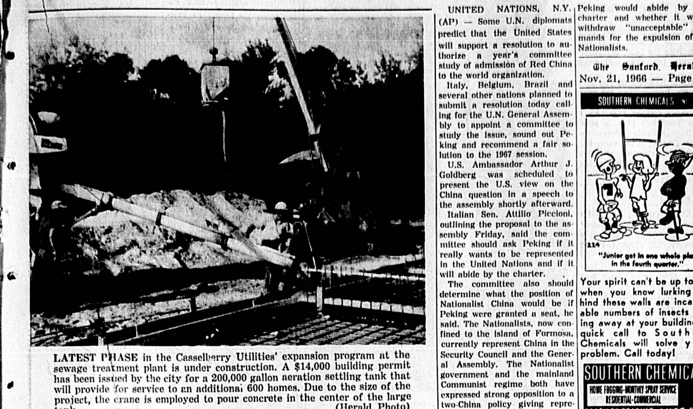
LATEST PHASE in the Casselberry Utilities' expansion program at the sewage treatment plant is under construction. A $14,000 building permit has been issued by the city for a 200,000 gallon aeration settling tank that will provide for service to an additional 600 homes. Due to the size of the project, the crane is employed to pour concrete in the center of the large tank. (Herald Photo)
