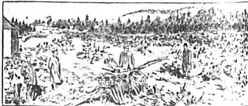
Drawn from actual photograph. Stumps blasted out into the ground.
