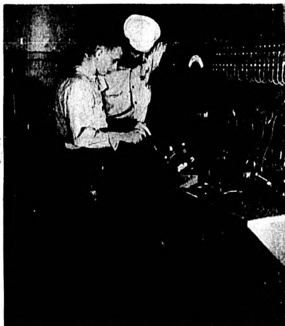
Working at the magneto test stand in the accessory shop of FASRON 821, Chester Duane Pruitt, AN, USN (left) and Ihon Zarinski, ADE1, USNR, run a check on a magneto.
