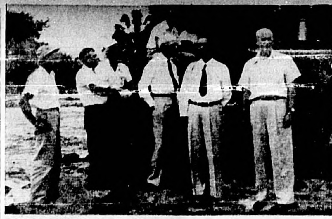
SANITARY LAND-FILL—Recently a delegation of city officials from Savannah, Ga., asked Sanford's manager, health officer and members of the Savannah Chamber drove to Sanford and inspected this city's model land-fill. City Manager Warren Knowles, who is on the tractor, explained how Sanford overcame its problem with the assistance of James Hume. (Third from left) Sanford sanitation officer and Edgar Griffith, city superintendent of streets. (far left). (Staff Photo)
