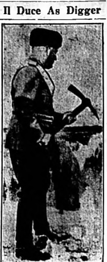
Premier Benito Mussolini is shown as he personally worked a patch in Rome, part of his comprehensive plan for reconstructing the city to make it more habitable and beautiful. (Associated Press Photo)
