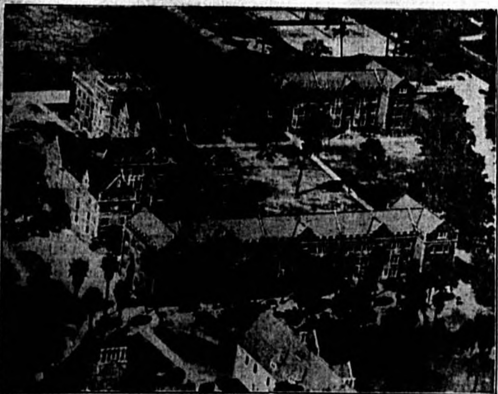
THREE NOW, BUT A FOURTH IS GOING UP—University of Florida's entire dormitory facilities are shown in this aerial view, but construction has begun on a fourth dormitory which will give the state university accommodations for an additional 230 students. At the present time the dormitories provide for only 15 percent of the student body of over 3200. Thomas Hall, shown in the upper part of the photograph, was the first building erected on the campus when the state's system of higher education was reorganized and the university opened in 1905. The new dormitory now under construction will parallel the two present dorms, and at the upper end, will project to the east a short distance.
