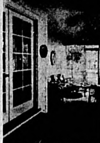
DOOR OF ponderosa pine opens off new rear porch.
