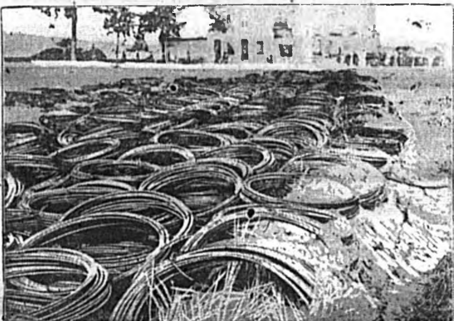
Photo copyright, 1914, by American Press Association. The Germans took thousands of coils of wire with them from Hamburg into France and used them as protection against artillery fire. The coils were placed in front of trenches to smother shells that fell in them.
