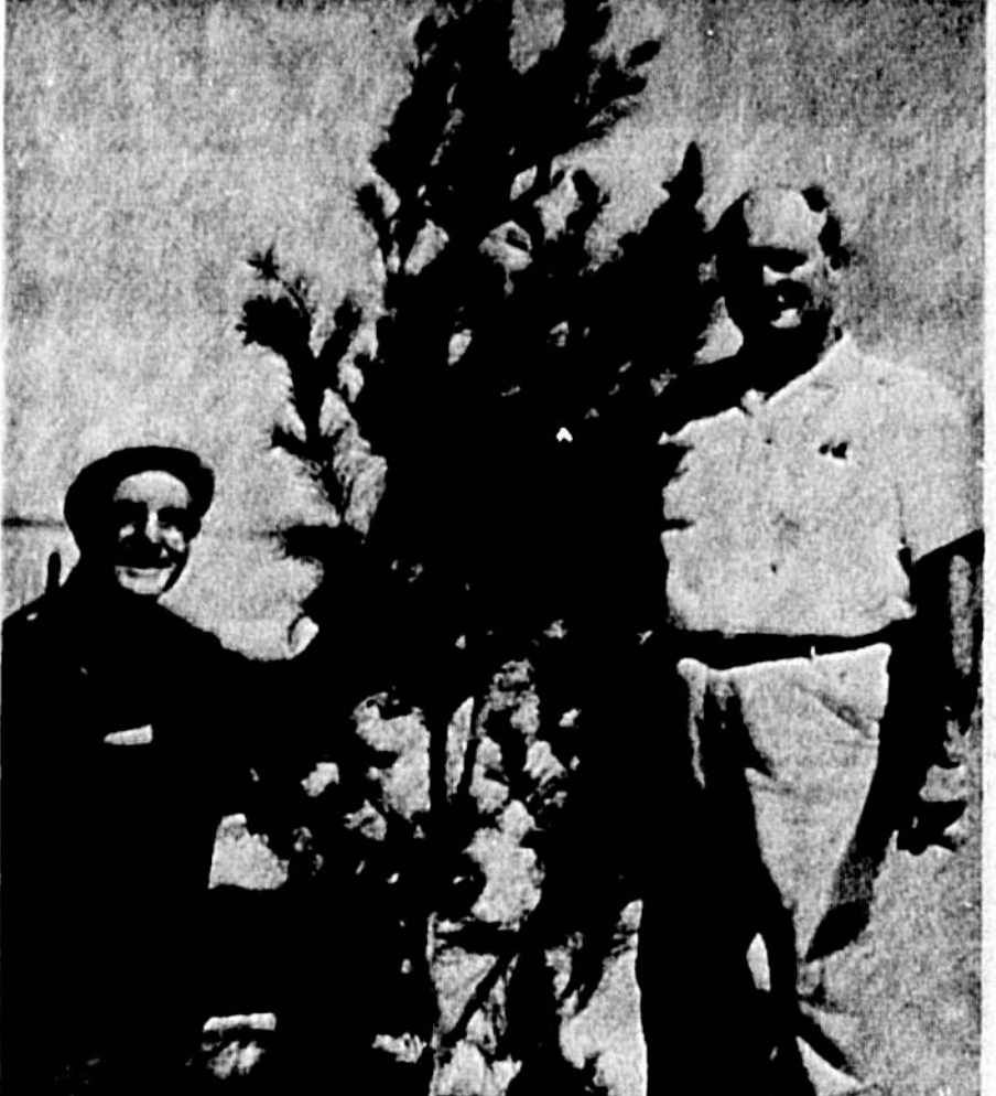
'TOPPING OFF' ceremonies for the Holiday Inn motel were held this afternoon with the traditional planting of a pine tree atop the structure on the lakefront.
