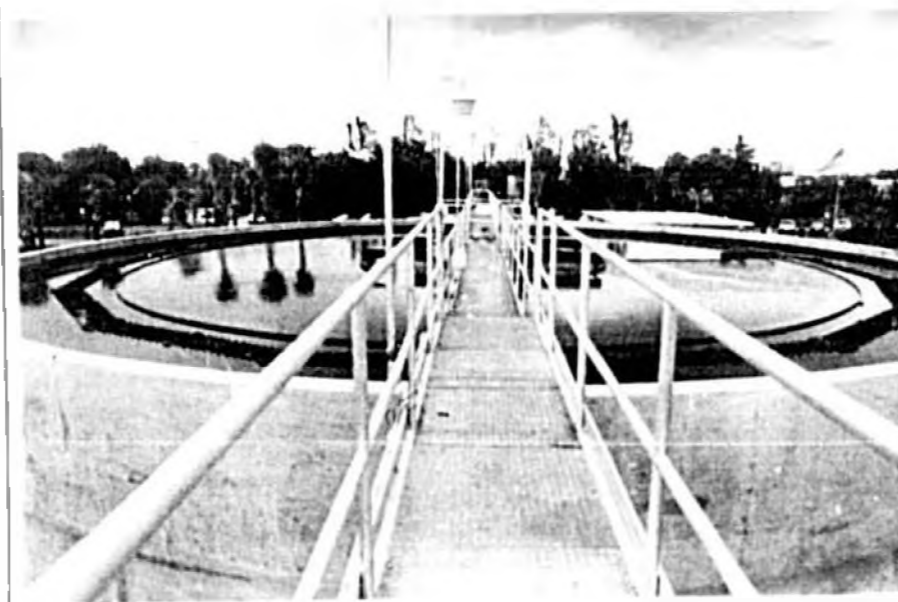
The new plant will be cleaned up Lake Mary, as well as provide for Sanford water supply.
