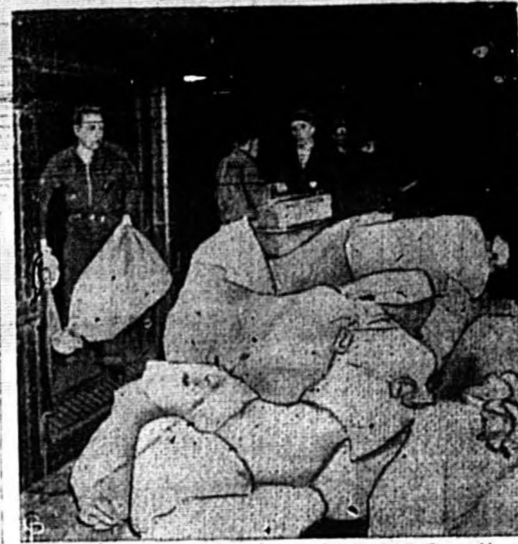
MAIL SACKS ARE UNLOADED during the fall strike at Pennsylvania Station, N. Y., shortly after their arrival from Philadelphia. The Post Office Department has imposed a nation-wide embargo on all but first class and air mail for delivery out of town. A weight limit of 16 ounces has been fixed on each piece to be carried off town. (International)
