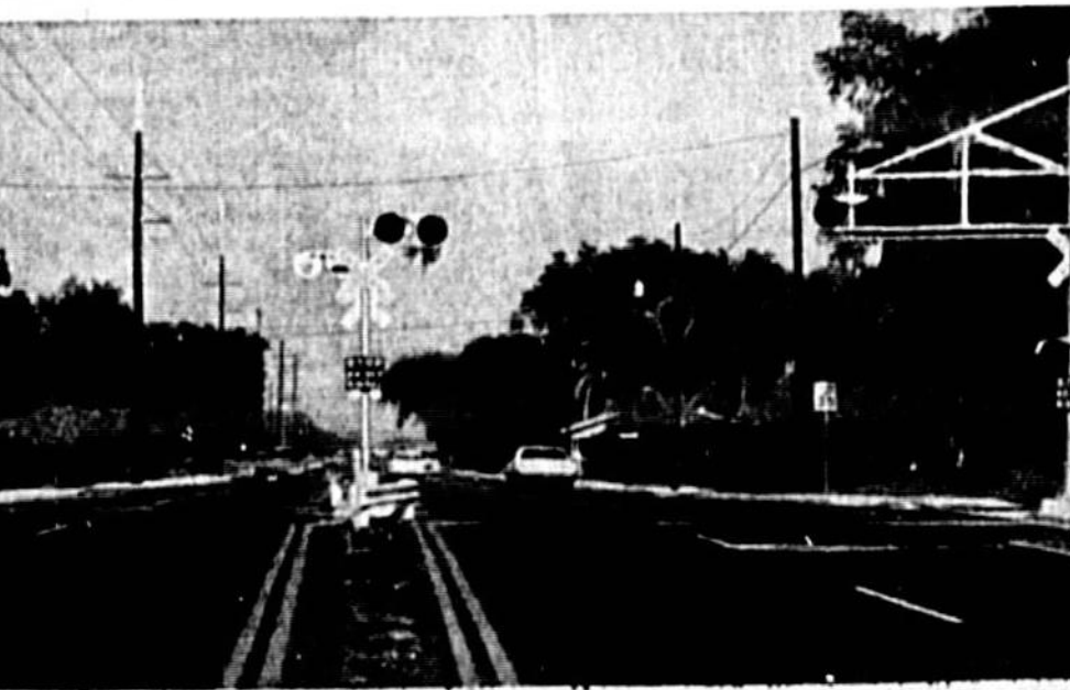
CONTROVERSIAL RAILWAY SIGNAL TO REMAIN IN ROADWAY... if city commission accepts compromise plan offered
