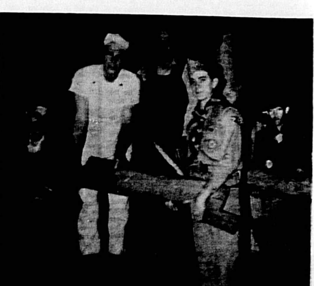
REPAIRS on the Lake Mary Boy Scout Hut are being made in response to request issued by Al Case, institutional representative, at monthly meeting of the Chamber of Commerce, sponsor of Troop 242. Scouts Robert Reed and Charles Frye are shown assisting volunteer workers (from left) Wesley Ricker, Homer Gleason and Arthur Brackett. (Photo by Violet Beckhorn)
