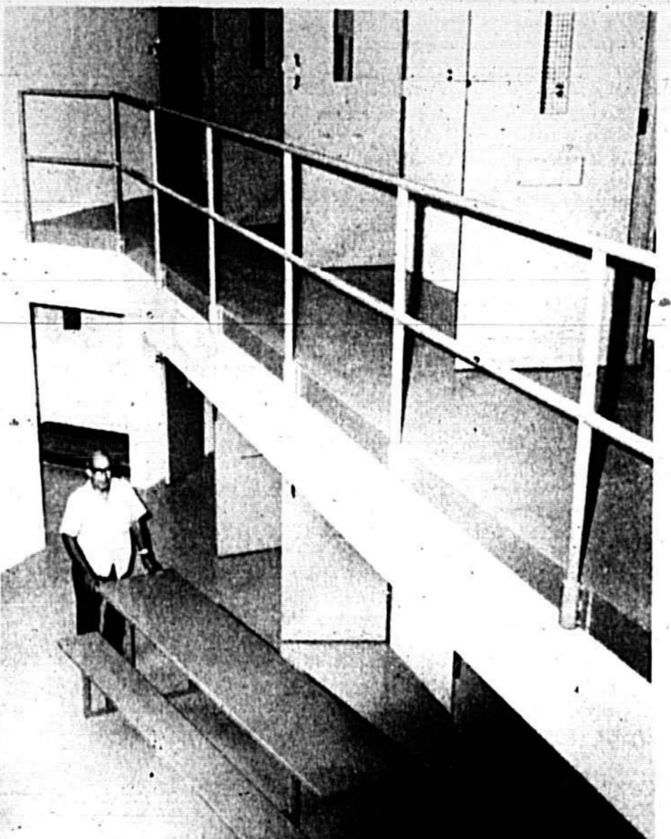
A worker positions a table in the inmates' public area in one of the jail's two-tier cell blocks. The division of the jail into three pods of four independent blocks each will allow prisoners to be "classified" and separated into groups by crime, age and behavior.
