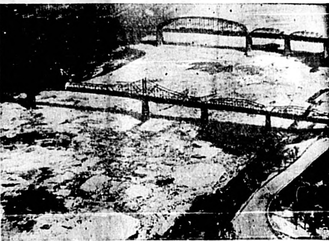
THIS AIRVIEW OF THE ICE-CHOKED Ohio River shows the ice jam which formed at Cincinnati causing $100,000 damage and threatening flood conditions. Ice clogged twenty feet high in some places and jammed at Ludlow, Ky., with the river rising six inches an hour. Shown above are the L. & N. Bridge (background) and the Central Bridge (foreground) with the public landing dock between them. In the foreground is the new flood wall being constructed in Kentucky. One boat was reported to have been sunk. (International Soundphoto)
