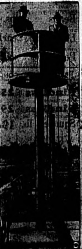
Rises by hydraulic lift this new tower at Santa Anita hotel. Presiding Steward C. J. Fitzgerald, left, and William A. Quigley to a vantage point 20 feet high during a race. Then the tower sinks back to the ground to give spectators a clear view of the tote board.
