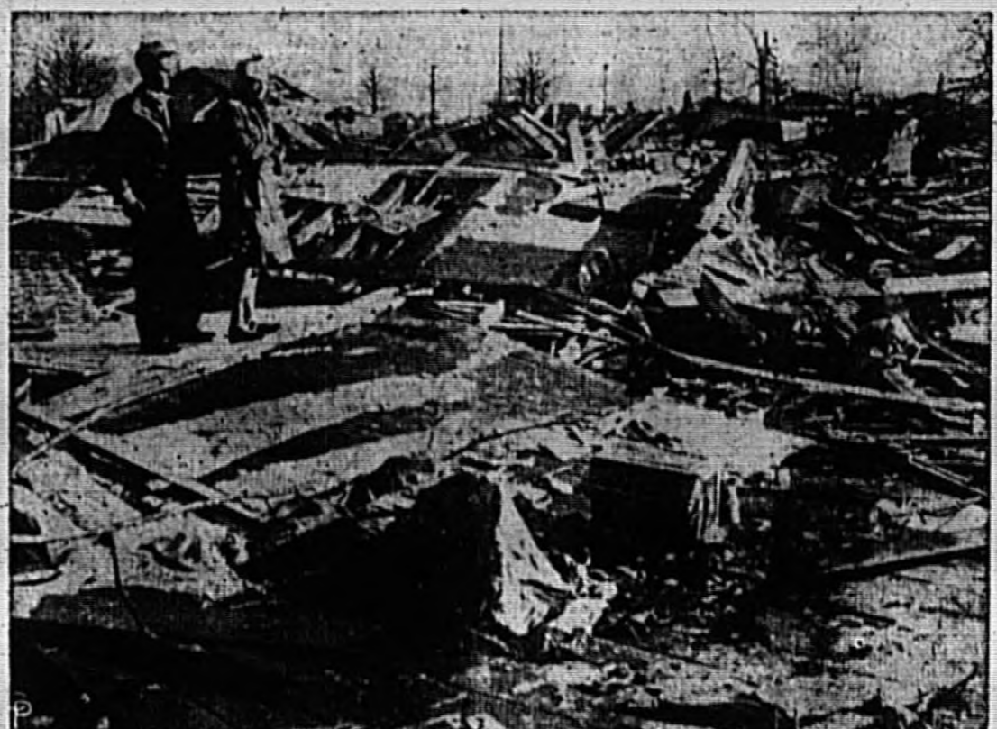
Mr. and Mrs. W. L. Thompson stand amid wreckage of their home in Cotton Valley, La., prosperous oil town which was virtually demolished by tornado. At least 25 persons were killed and hundreds injured or made homeless by the storm. (International Soundphoto)
