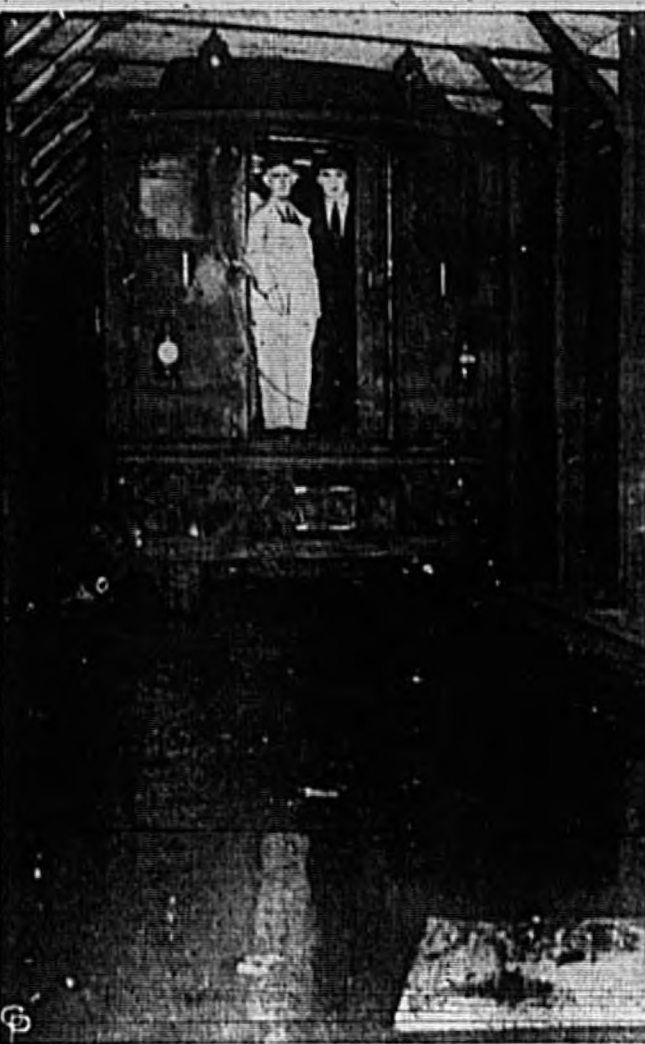
A BREAK IN A 36-INCH water main on New York's West Side brings a subway train to a halt on the IRT line at 80th Street and Broadway. Nine thousand passengers were trapped for a short time when water poured into the tunnel. Service was suspended 5 hours. (International)
