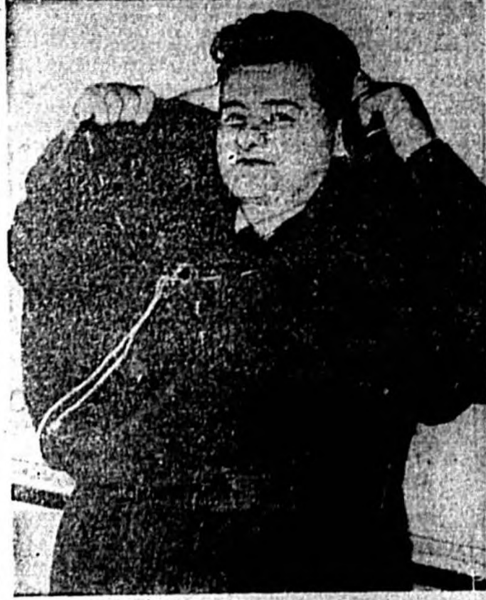
Capt. Erling Vorberg, of the torpedoed Norwegian tanker Barforn , poses in one of the rubberized overall-type life saving suits used by some of the members of his crew when the tanker sank. He declared the boatswain floated unconscious in the suit until help came. Heavy boots keep the wearer in an upright position.
