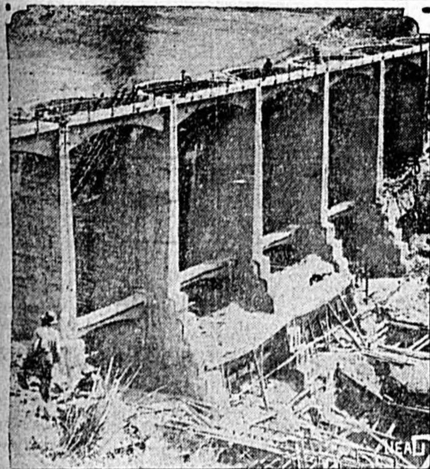
Salt Lake City is more than usually interested in the condition of this dam, which some engineers declare unsafe. It is under construction at Dell Mountain, Utah, 16 miles from Salt Lake City, and if it should collapse it would turn 600,000,000 gallons of water on the city. New tests of its strength are being made.
